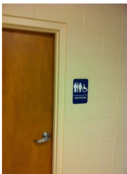
ADA Compliant Toilet Room
