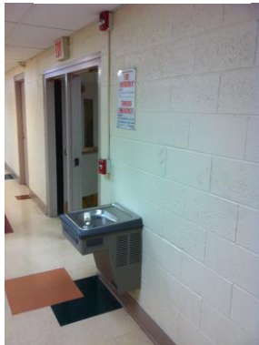
Accessible Drinking Fountain and Visual Fire Alarm Strobe above.
