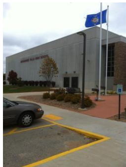
Gym at south west side
