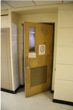
Typical classroom door
