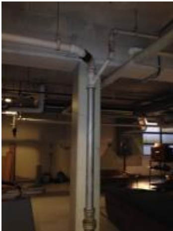
Original Sanitary Piping
