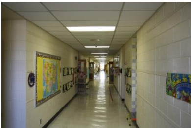
Second floor hallway ceiling tile
