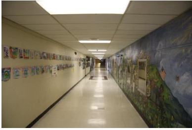
CMU corridor walls / VCT flooring
