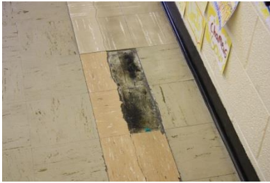
Damaged 9"9" VCT tile on second floor
