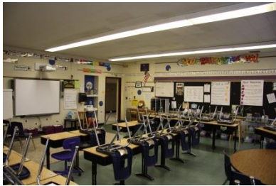
CMU Classroom walls
