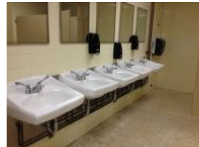
Lower Level Toilet Room: New Lavatory Fixtures
