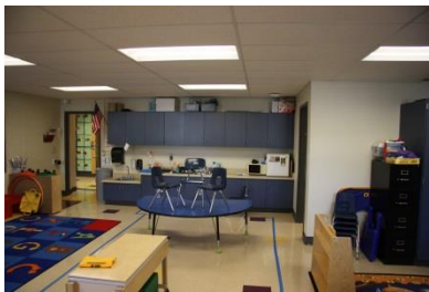
Drywall classroom walls/ VCT flooring
