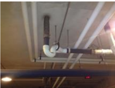
Repaired Sanitary Piping
