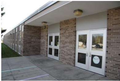
Playground drainage issues
