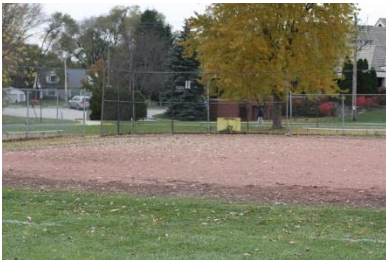
Rusting baseball field fence
