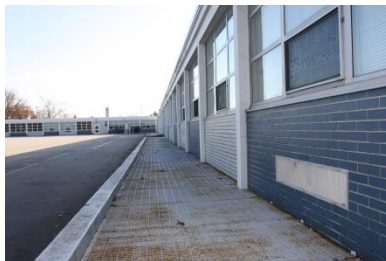
Window well grate
