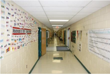
CMU corridor walls / VCT flooring
