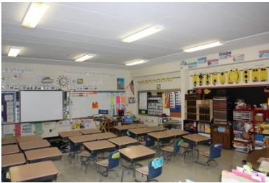
CMU Classroom walls
