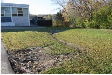
Playground drainage issues
