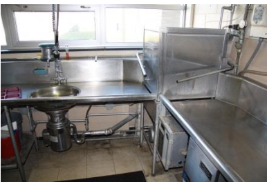
Damaged VCT flooring in kitchen
