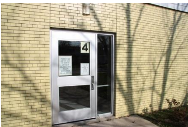
Typical exterior door
