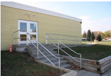
Ramp at Northwest stairwell
