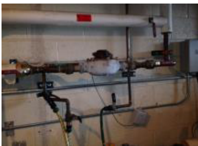
Irrigation Water Meter
