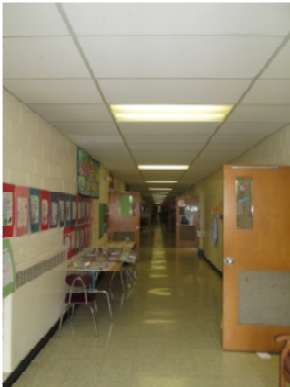
Concrete block corridor wall/ VCT
