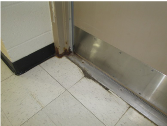
Rusted hollow metal door frame
