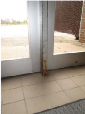
Rusted hollow metal door frame
