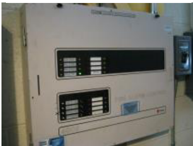
Fire Alarm Control Panel
