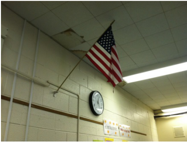
Stained / damaged ceiling tile
