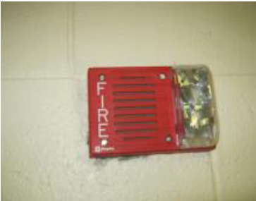
Fire Alarm Notification Appliance
