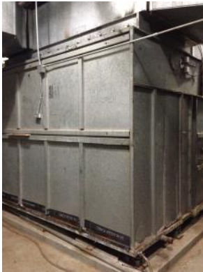
Multi-Zone Air Handling Unit
