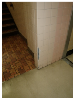
Damaged wall tile
