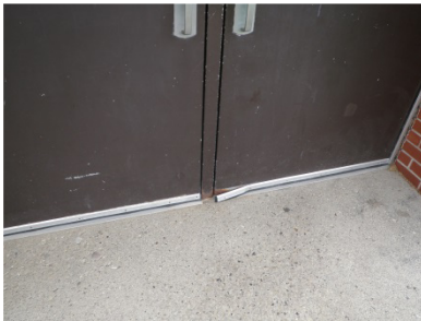
Damaged weatherstripping
