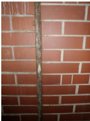
Deteriorated control joint
