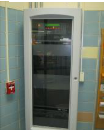
Fire Alarm Control Panel
