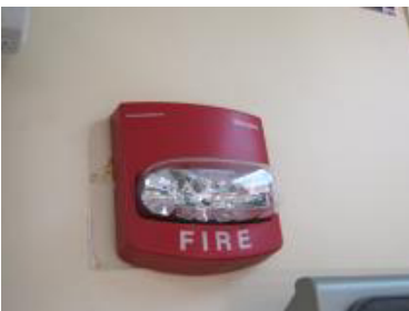
Fire Alarm Notification Appliance
