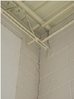
Cracked concrete block wall
