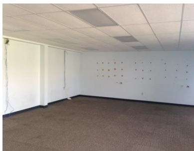
Typical drywall walls
