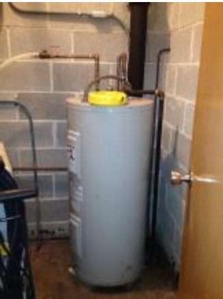
Electric Water Heater
