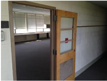
Typical classroom door
