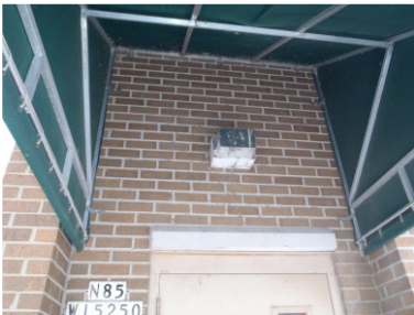
Canopy at main entrance
