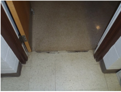
Stained / damaged ceiling tile
